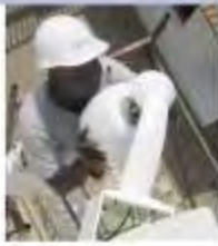
A Westminster engineer installing surveillance equipment in West Africa
